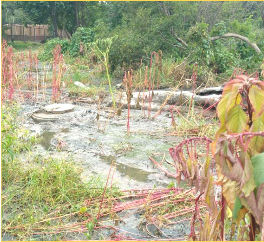
■ Sewer blockage - Fourways, July 2017
